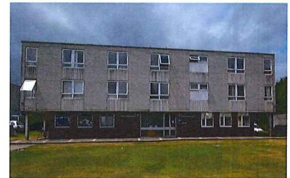
Plymouth House (Residential Plot A) at Middlemoor, Exeter, which is on land to be redeveloped for reinvestment examples of reducing demand on the estate
